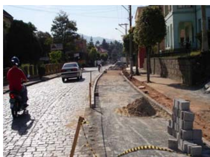
The cycle way under construction
