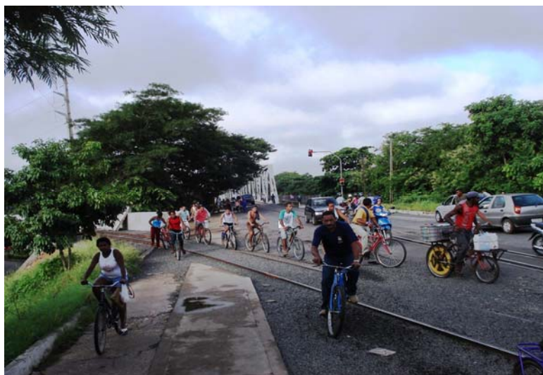
Commuter cyclists crossing the railway that cuts the cycle way at this point
