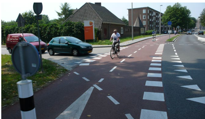
Safe crossing of a one side, two directions cycleway at side road (Arnhem, Netherlands)
