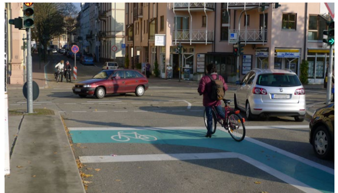
Bicycle box for safe turning left (Offenburg)
