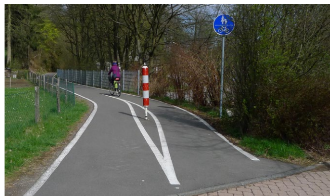
Visual contrast at bollard to prevent one-sided accidents (Cologne region)
