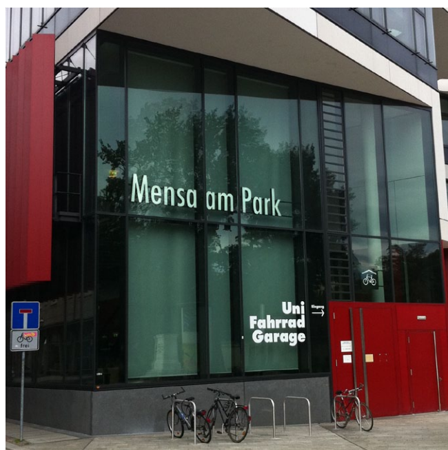
University restaurant in Leipzig: Parking facilities for short duration on the street and for longer stays in the garage. © Sebastian Korn
